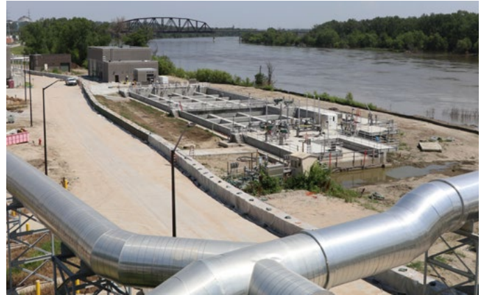
Aerial view of wet weather chlorine contact basin under construction at the MRWRRF, CSO 102.
